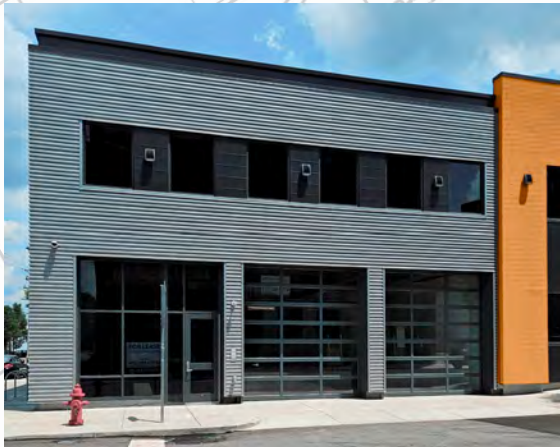
1ST FLOOR STOREFRONT GARAGE DOORS
