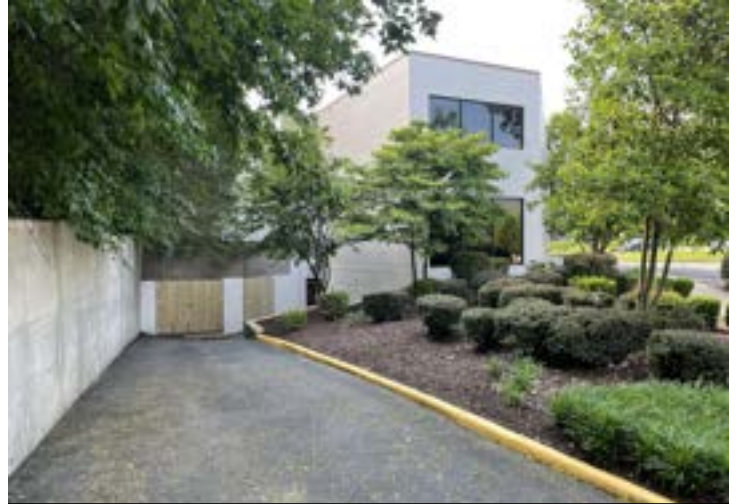
Front of Building and Loading Zone
