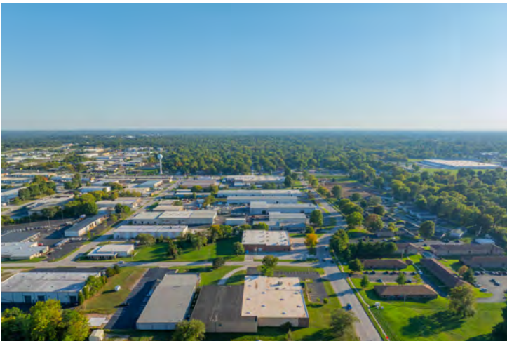
North Side Looking South
