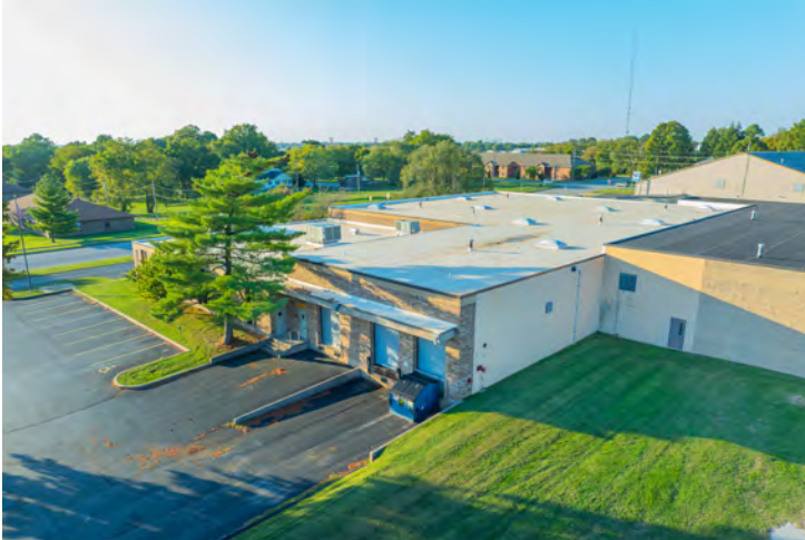
Southeast Looking Northwest
