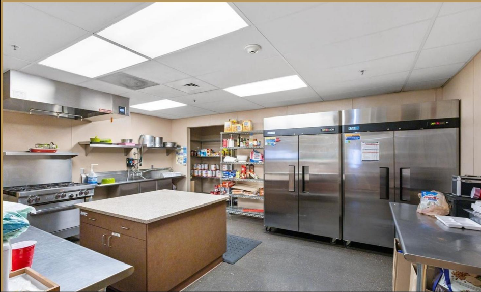
Commercial kitchen infrastructure
