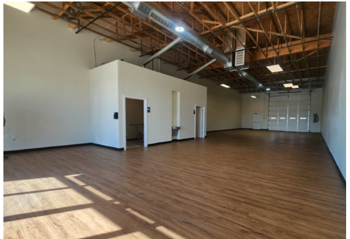
Typical Open Showroom
