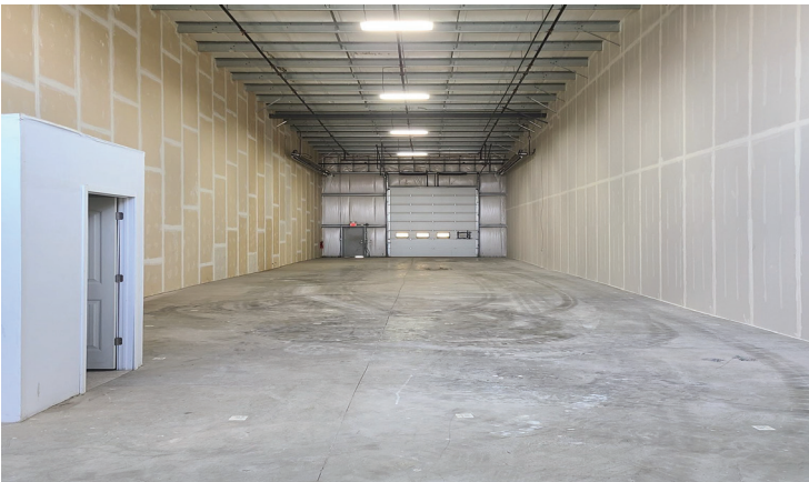
Bay prior to construction
