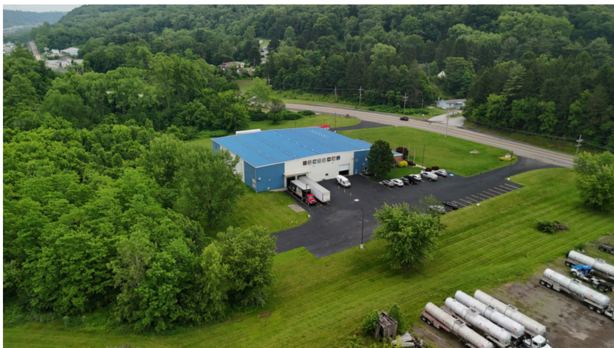
AERIAL VIEW — BUILDING LAYOUT & SITE ACCESS
