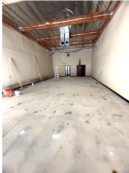
Warehouse this one is a single unit like #1, #2 and #7. 5-6 is a double unit.
