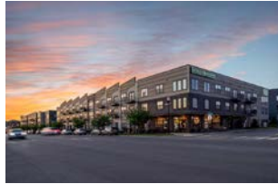
BEXLEY SILO BEND 193 APARTMENTS
