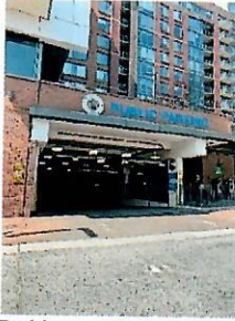
Parking garage behind the bldg.
