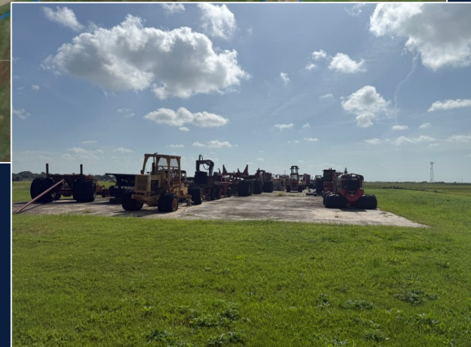
Concrete pad – equipment storage, work area or foundation for building
