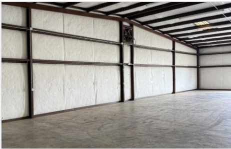
INSULATED CLEAR-SPAN BAY
