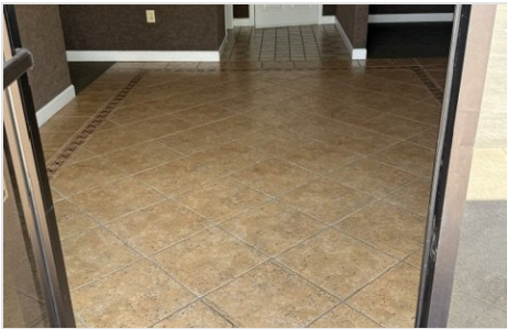
FINISHED OFFICE INTERIOR
