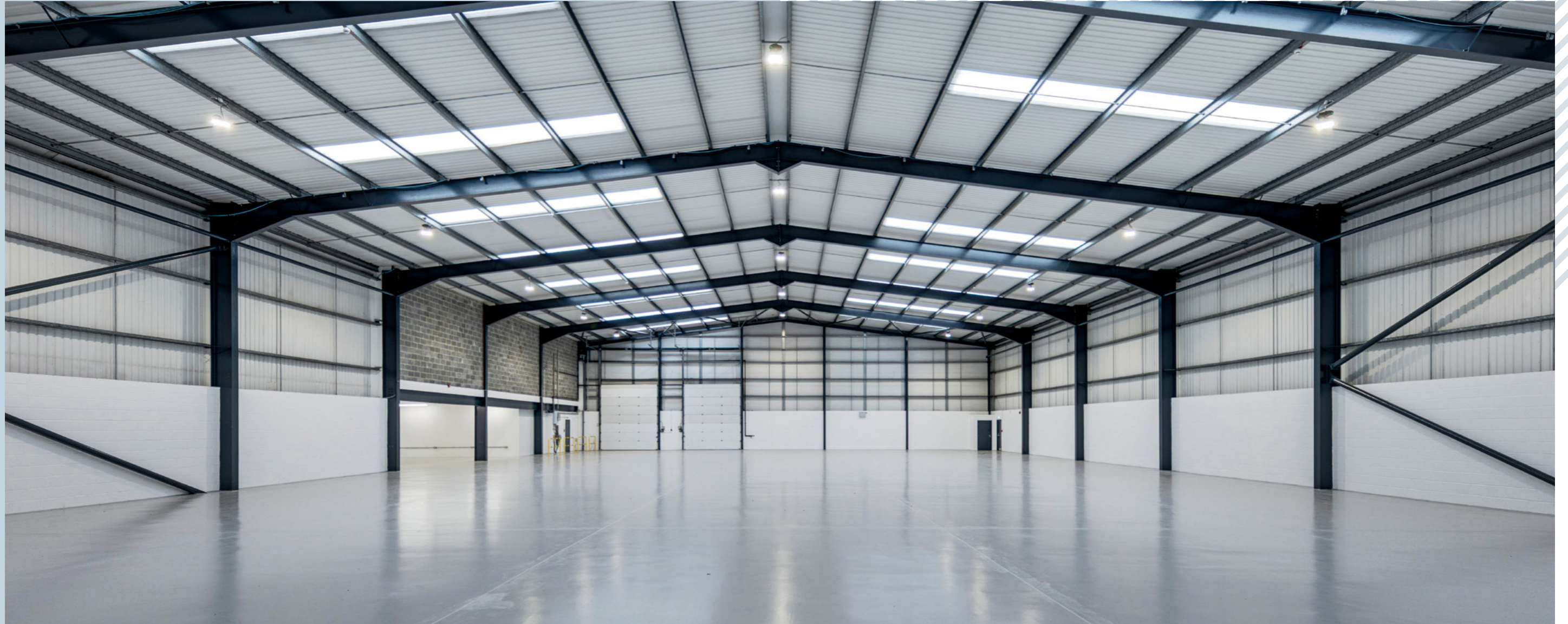
7.64m clear height & 2 electric loading doors
