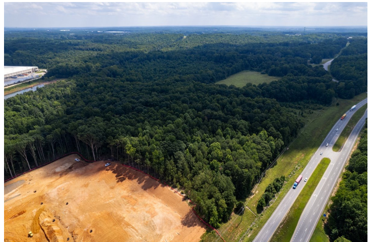
Adjacent construction site & Hwy 129
