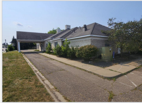
Covered entry with drive-through canopy
