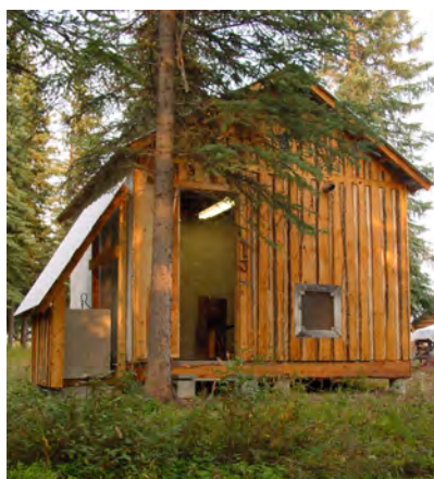
Back-up Generator Bldg, straw bale at 3 sides with framed 4th wall
