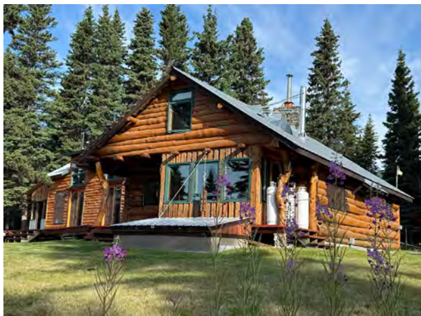
South face Lodge and battery vault
