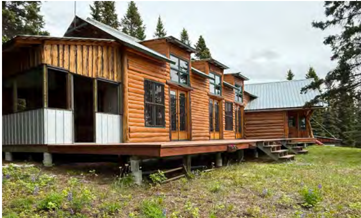
Deck & Lodge south face
