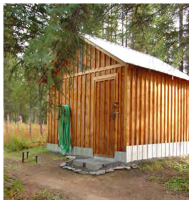
Pump House with 3 key boxes (lower left)
