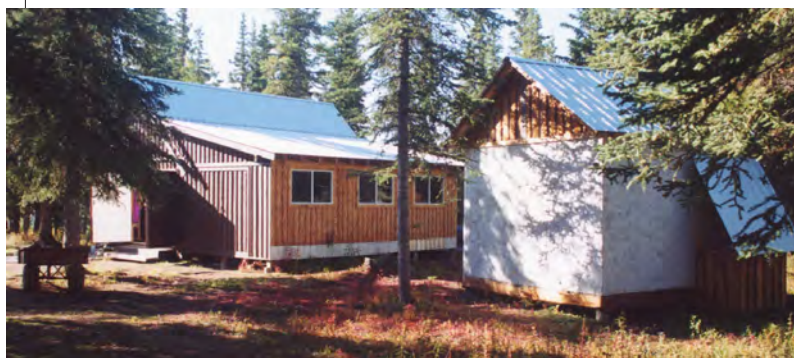
Shop and Back-up Generator Bldg
