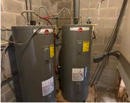
Rear Utility Room
