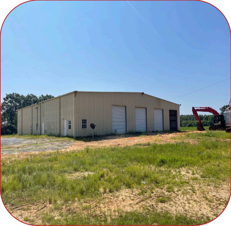
BACK FACADE | 4 ROLL UP DOORS
