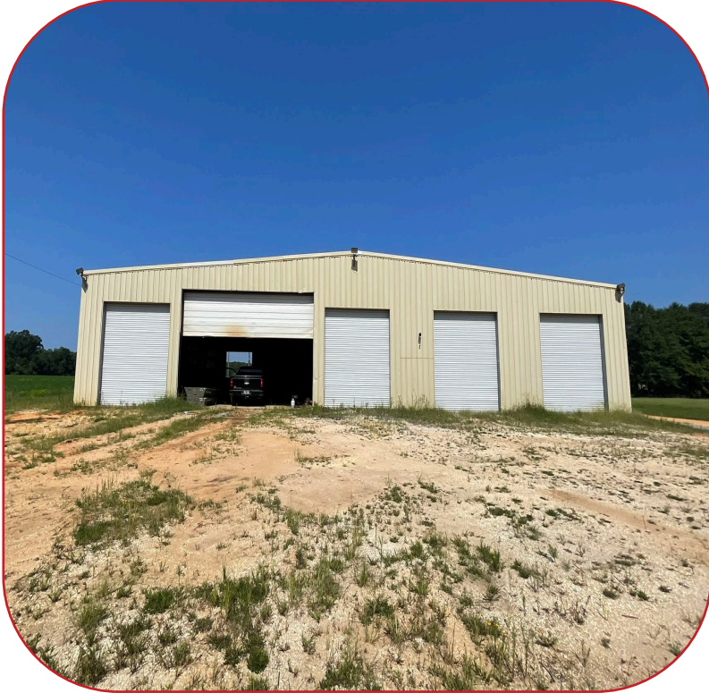
FRONT FACADE | 5 ROLL-UP DOORS
