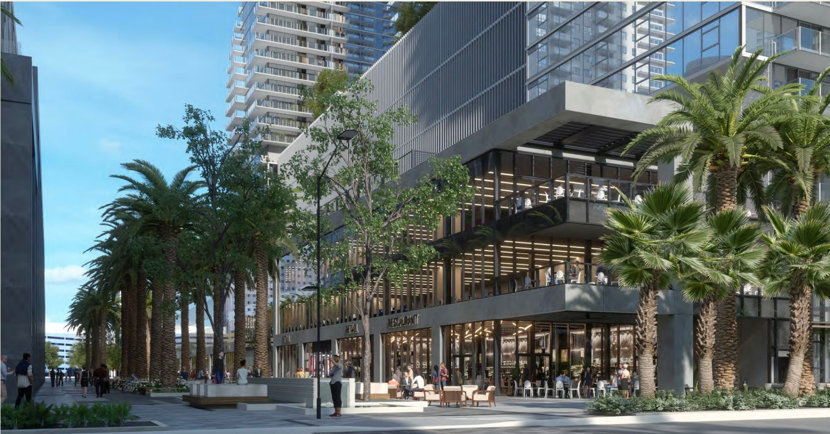
BLOCK E - East to West View
