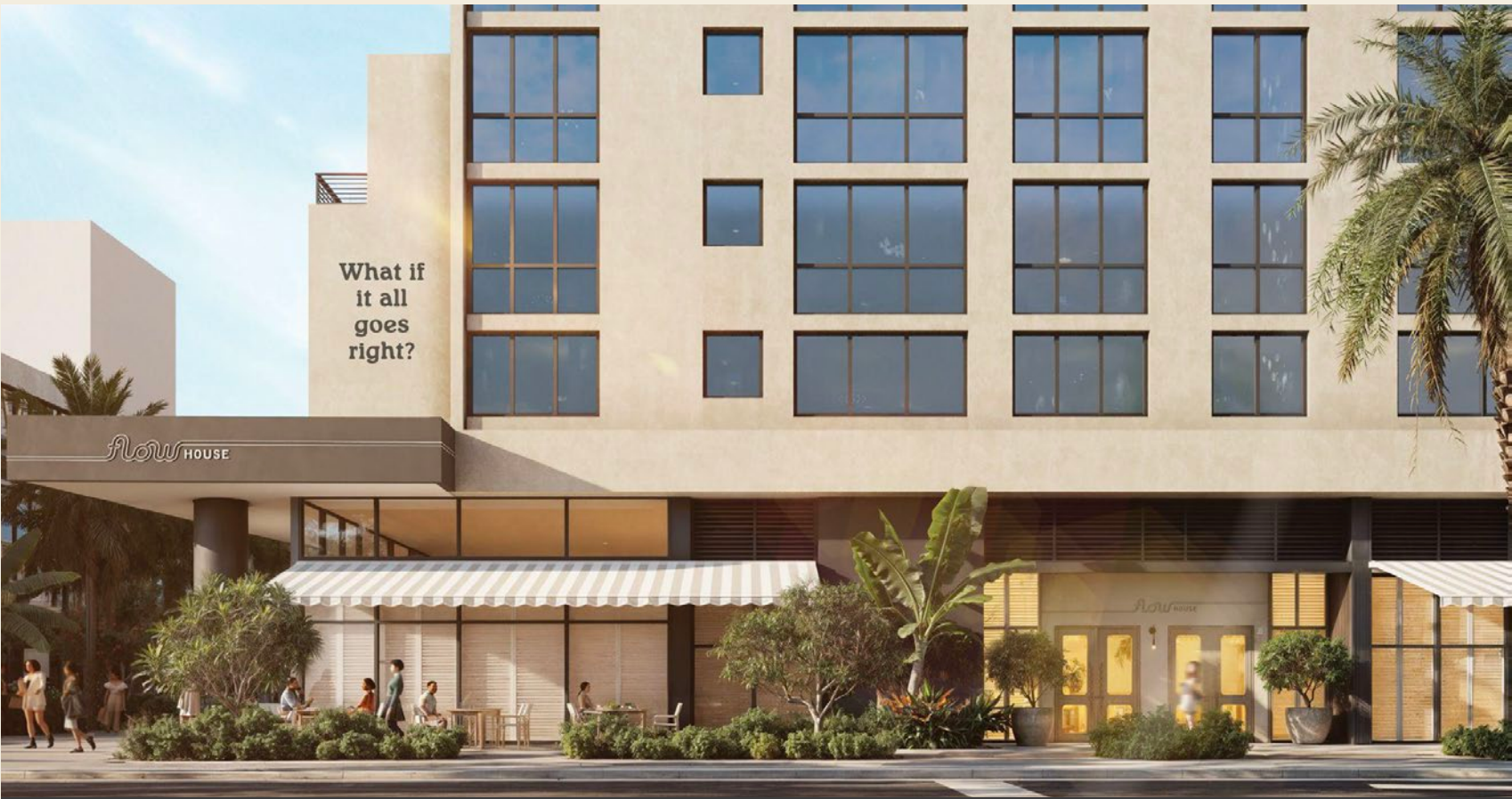
North Miami Avenue Facade
