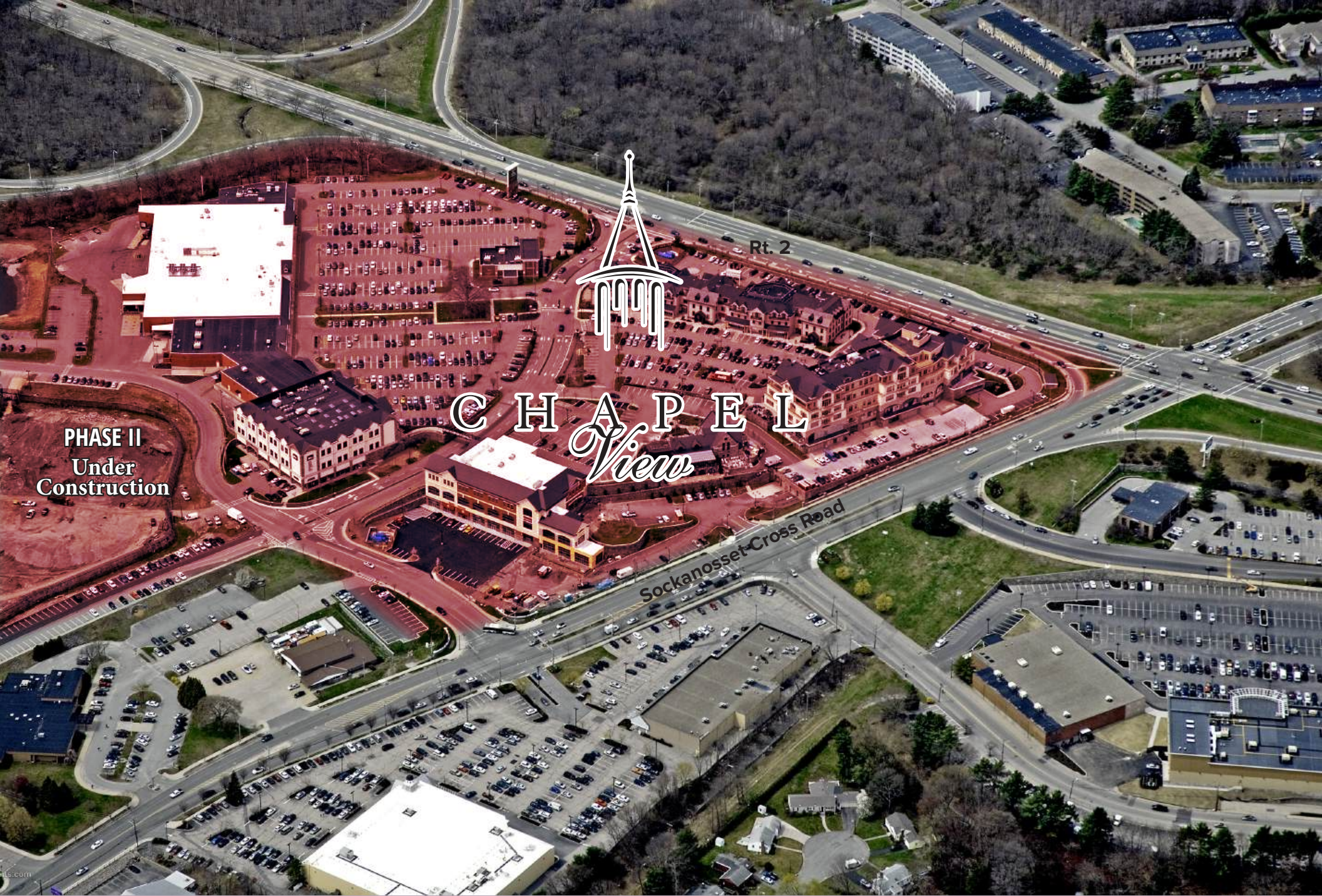
RI ROUTE 2 & SOCKANOSSET CROSS ROAD
