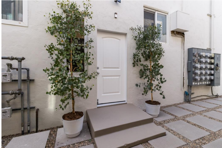
BRAND NEW EXTERIOR DOORS, WINDOWS, ALL NEW ELECTRIC METERS
