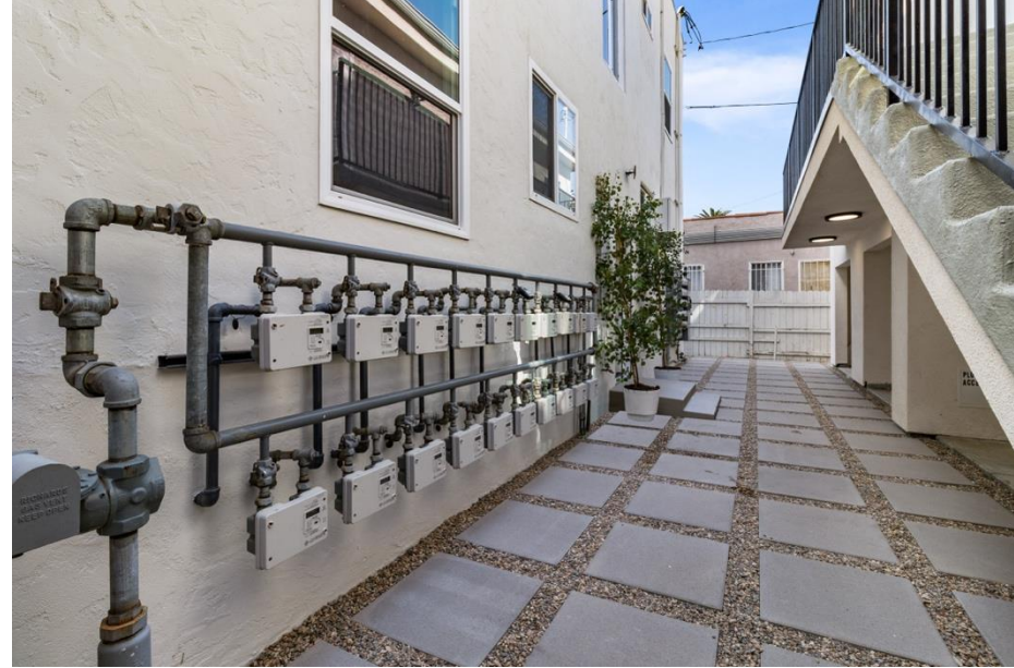
ALL NEW PLUMBING / ALL NEW GAS METERS
