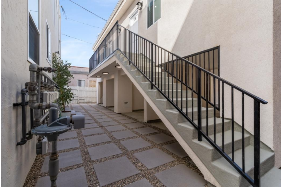
BRAND NEW GROUND UP CONSTRUCTION
