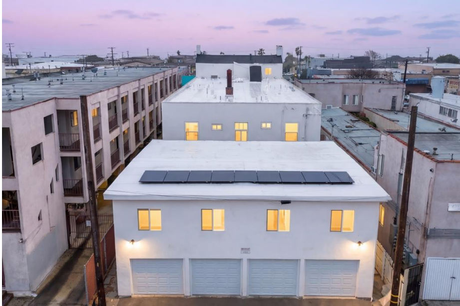
SOLAR PANELS ON NEW CONSTRUCTION, MECHANIZED GARAGES
