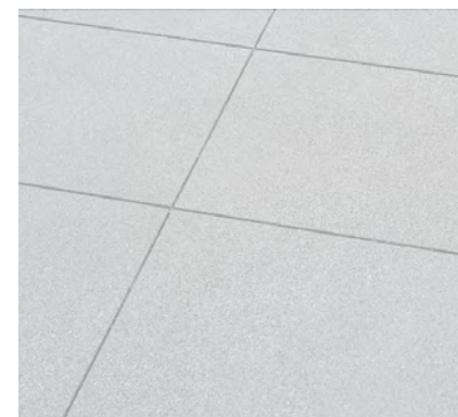
CONCRETE W/ SAWCUT JOINTS
