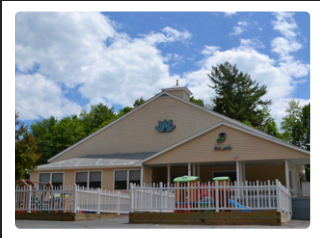
99 River St | Day Care Bldg.
