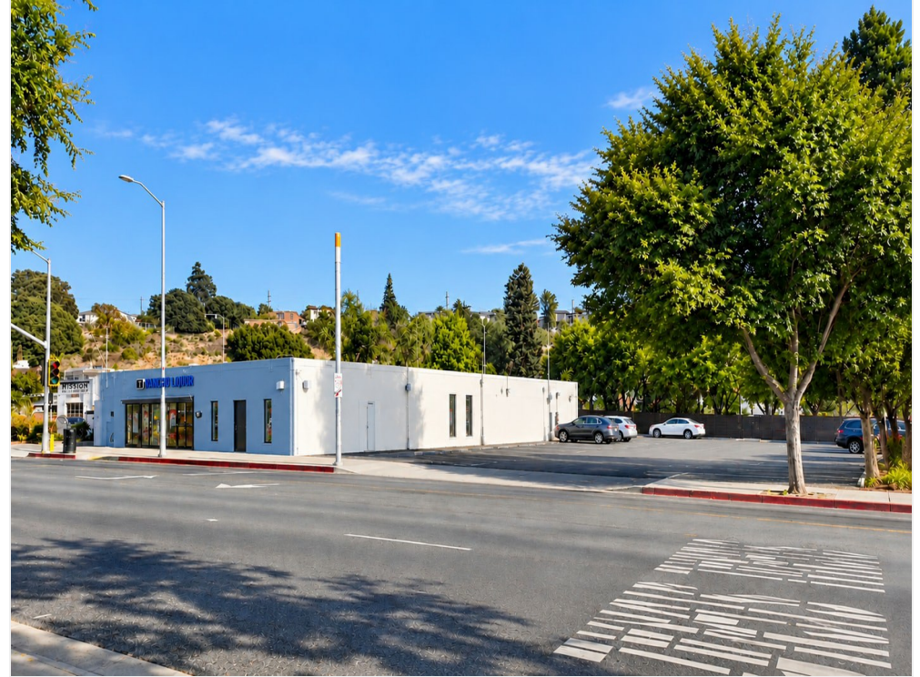
Front with Parking Lot
