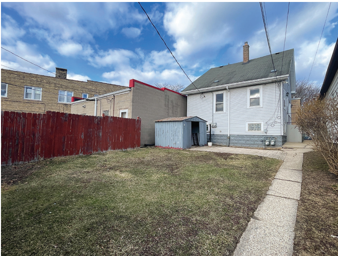
View of residential apartment unit and back yard.
