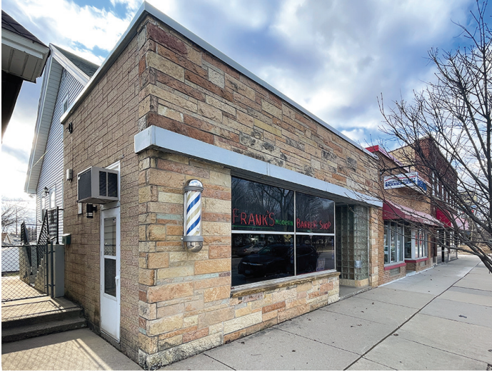
Commercial storefront with stone façade. Gated walkway on left leads to residential apartment (vinyl siding).
