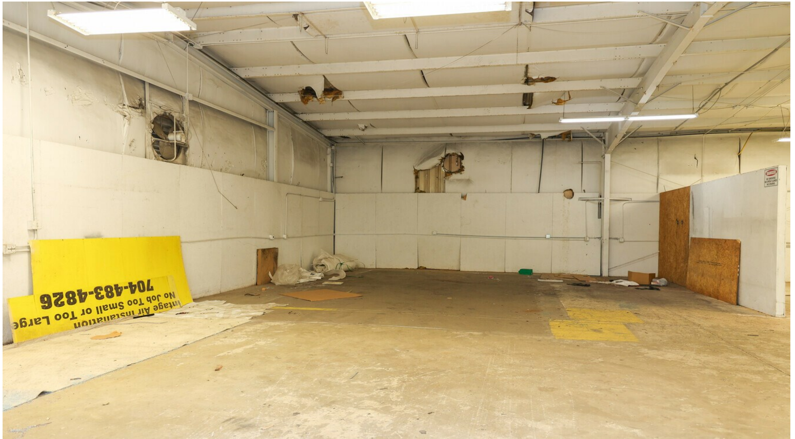
Alternate Warehouse View without Windows
