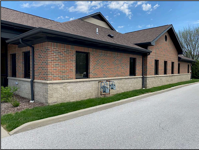
Subject space - Southern elevation
