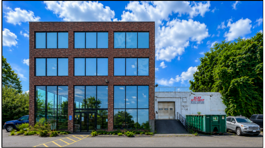
SIDE ENTRANCE TO SHOWROOM & DRIVE-IN DOOR
