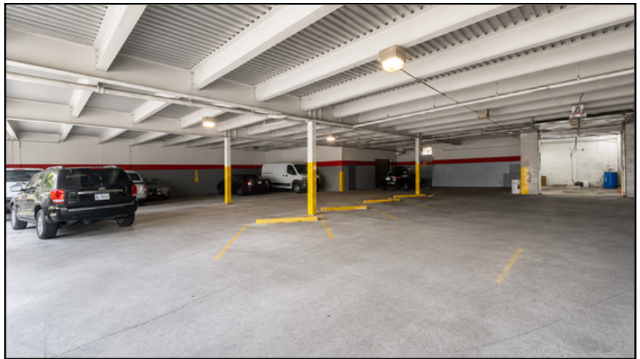
GROUND LEVEL PARKING GARAGE
