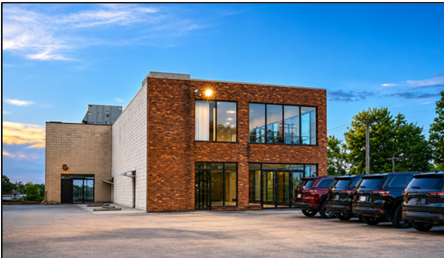
UPPER LEVEL PARKING WITH DIRECT ACCESS TO UPPER FLOORS
