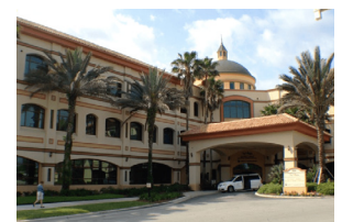
UF HEALTH HOSPITAL EAST
