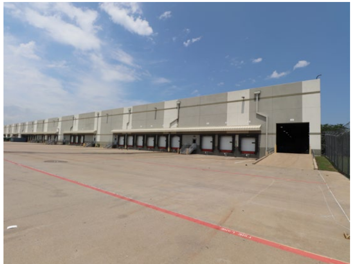
SOUTHWEST CORNER, FENCED TRUCK COURT
