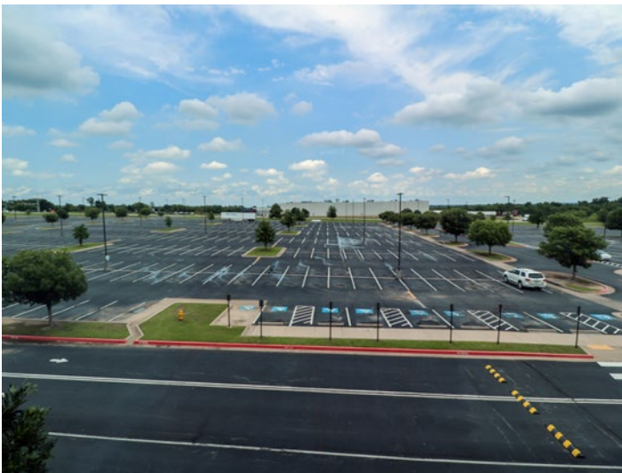
MAIN PARKING LOT
