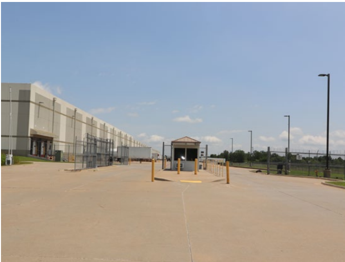
SOUTHWEST CORNER, GUARD HOUSE TO TRUCK COURT - TRAILER STORAGE
