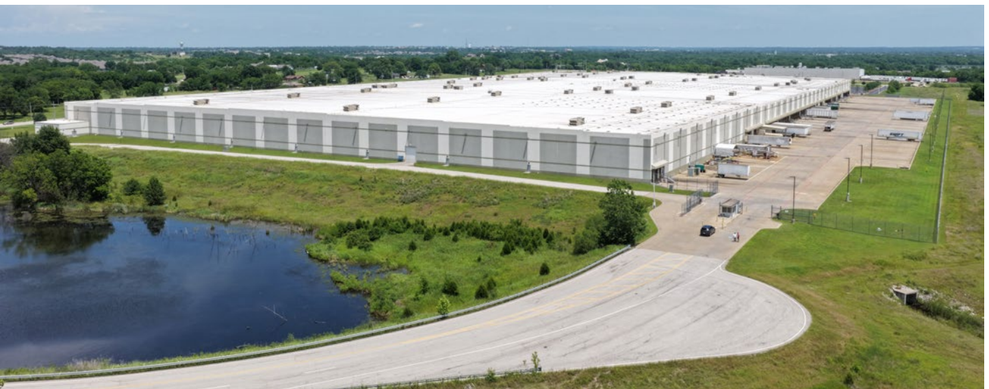
SOUTHWEST CORNER WITH GUARD HOUSE TO TRAILER COURT
