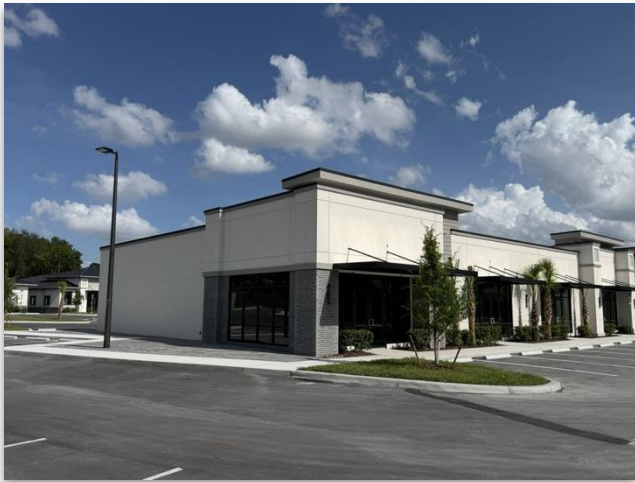
Storefront glazing along the frontage
