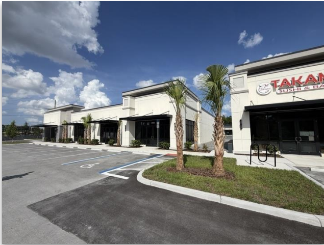
Corner approach from Ocoee Apopka Road
