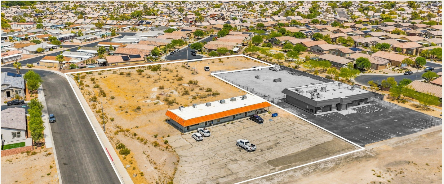
Aerial view — 2.2-acre site outlined, surrounded by established Henderson neighborhoods
