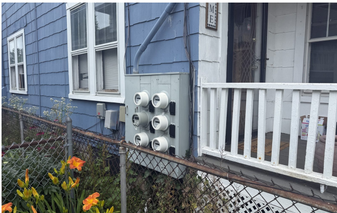
Separately metered — 6 electric meters
