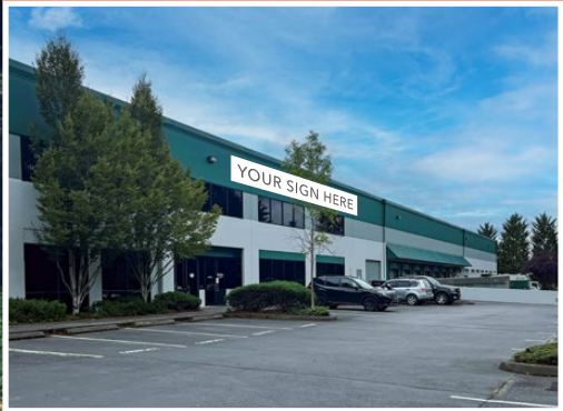
POTENTIAL FREEWAY SIGNAGE
