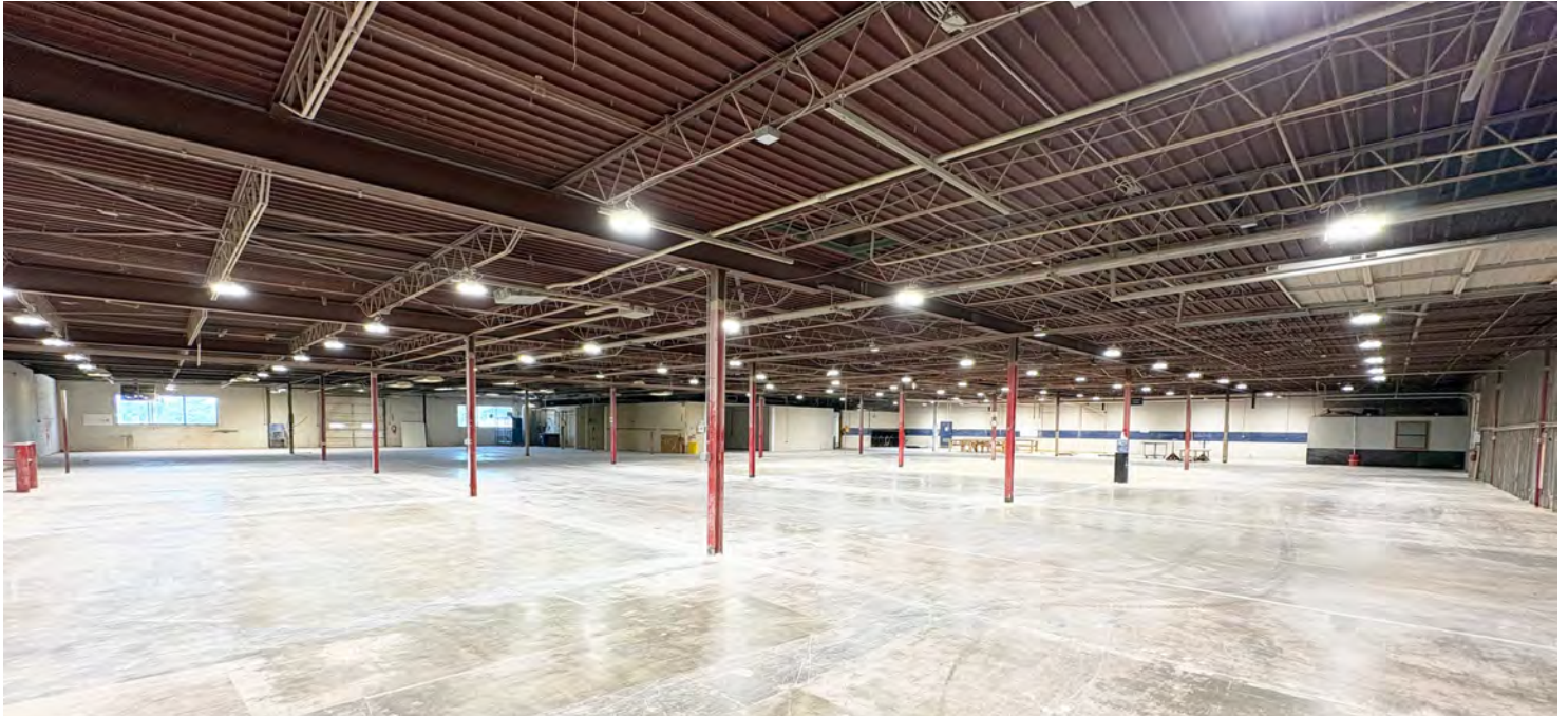
Interior of Warehouse
