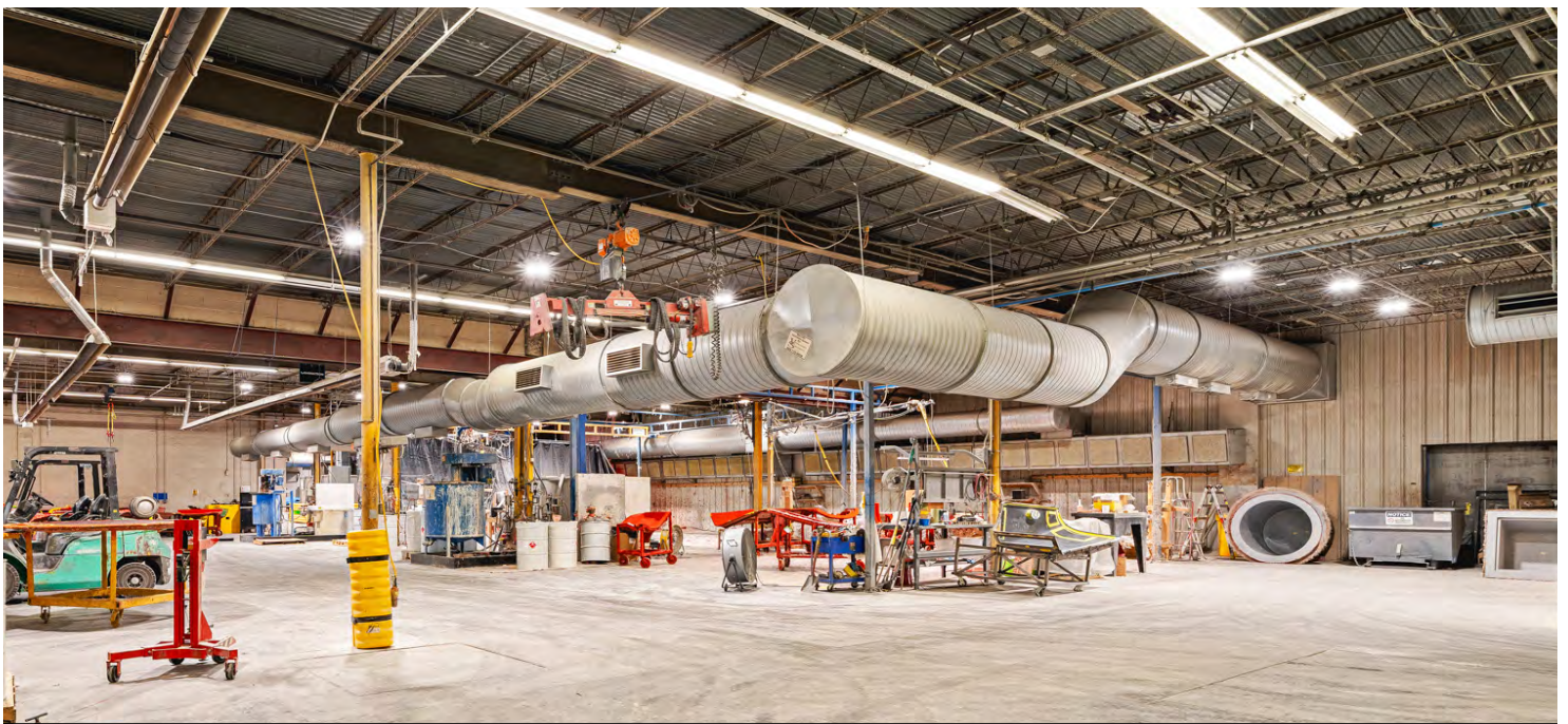
Interior of Warehouse
