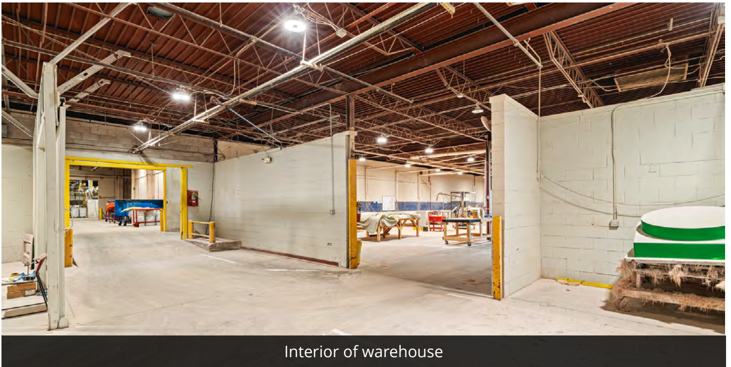
Interior of warehouse
