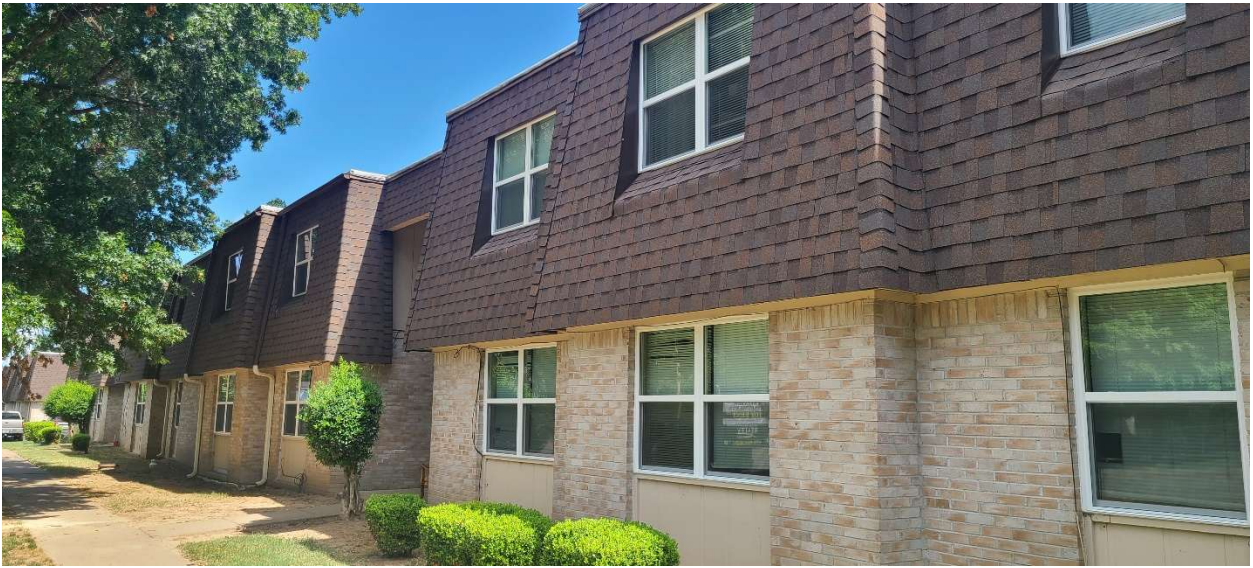
266 Windows were installed in July and August 2024. 50-year Roof Shingles installed in Dec. 2023.
