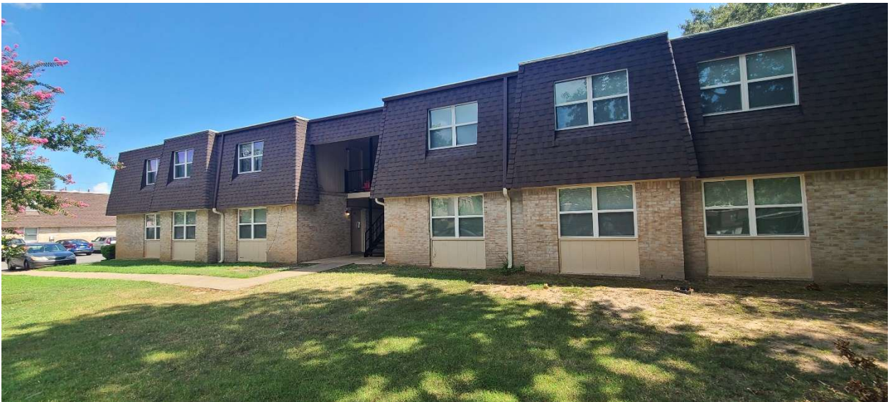
This is the smallest building which houses 8 units. The other 2 buildings house 16 units each.
