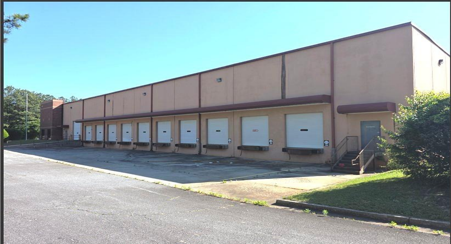
DOCK-HIGH DOOR ROW — 16 DOORS TOTAL
