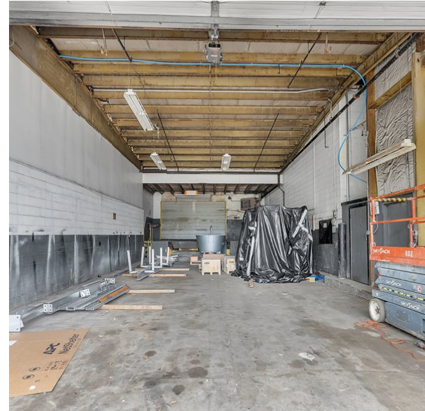
HIGH BAY WITH OVERHEAD HOIST
