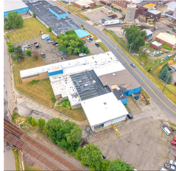
RAIL ADJACENCY · TRESTLE & YARD
