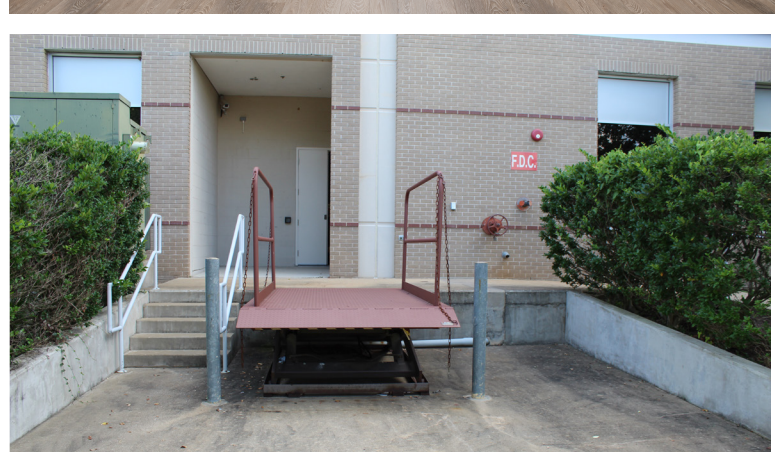
Loading dock capabilities
