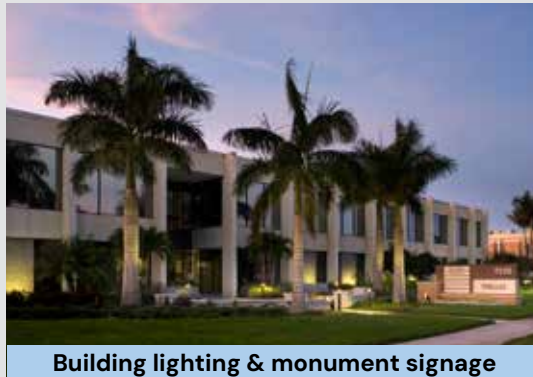
Building lighting & monument signage
