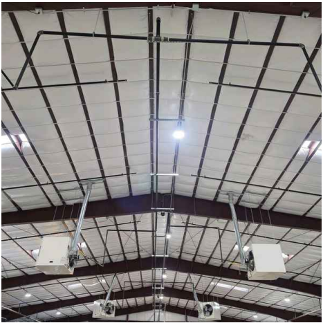
Ceiling Structure: Red Iron Beams
