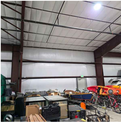
Wall Structure: Steel Columns
