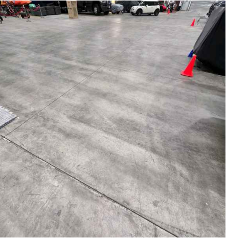
Foundation: Material Concrete, Slab on Grade
