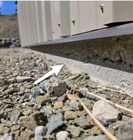
Foundation: Material Concrete, Slab on Grade
