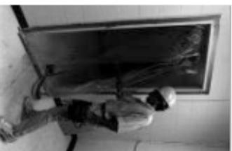
Close off entryways with an airtock.
