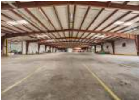
Building A warehouse
