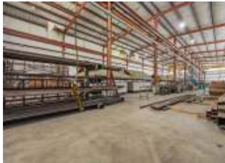
Building B steel shop
