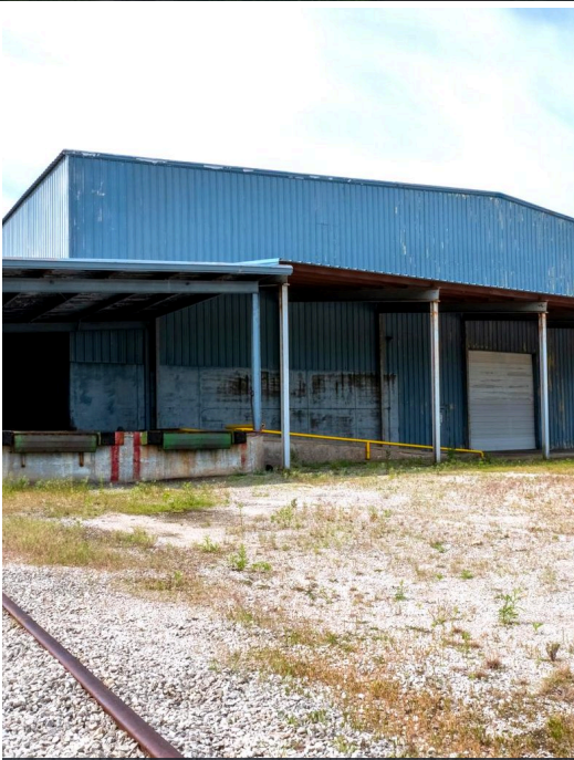
BNSF RAIL SIDING + DOCK
