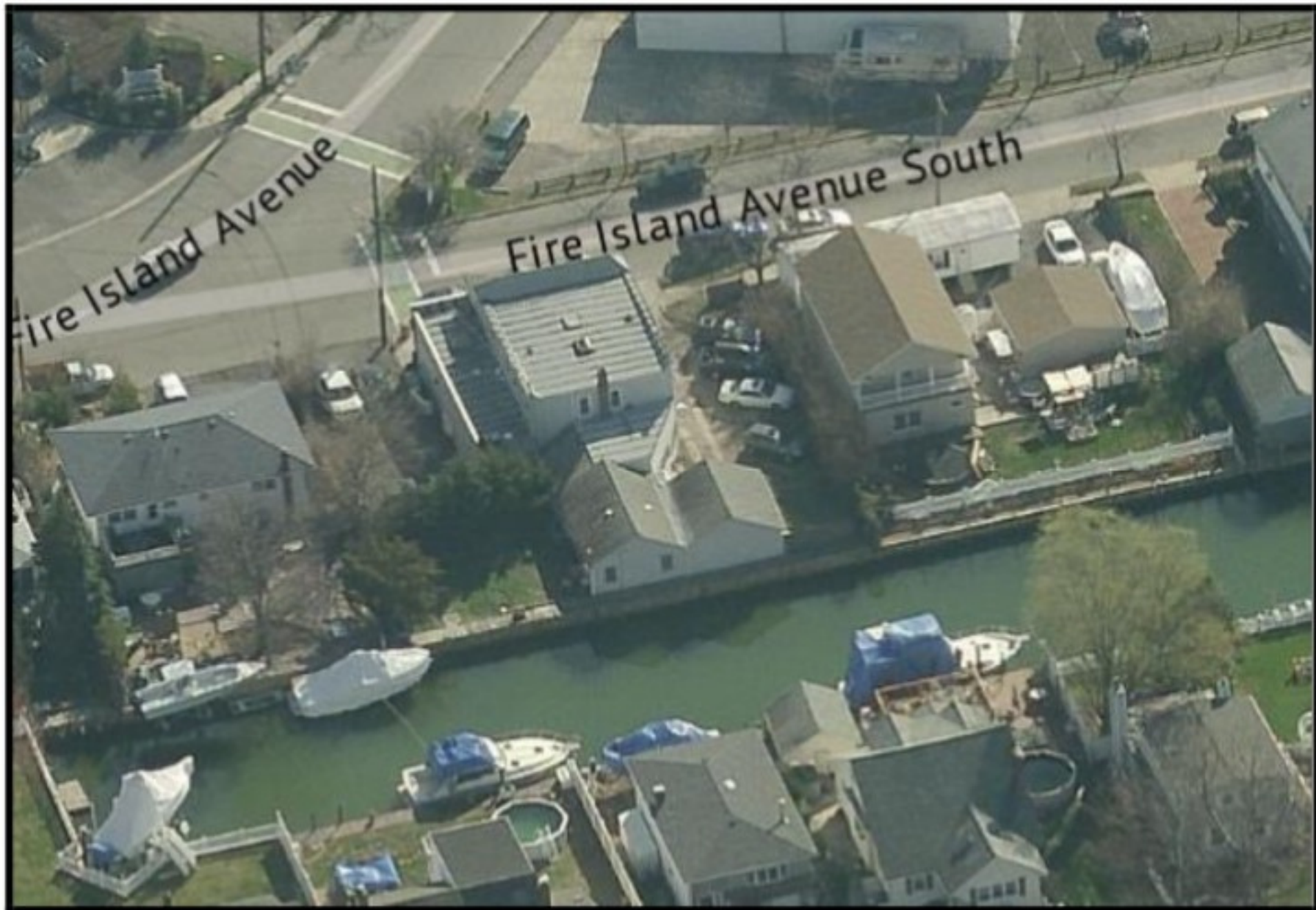
AERIAL VIEW FACING EAST FROM CANAL
