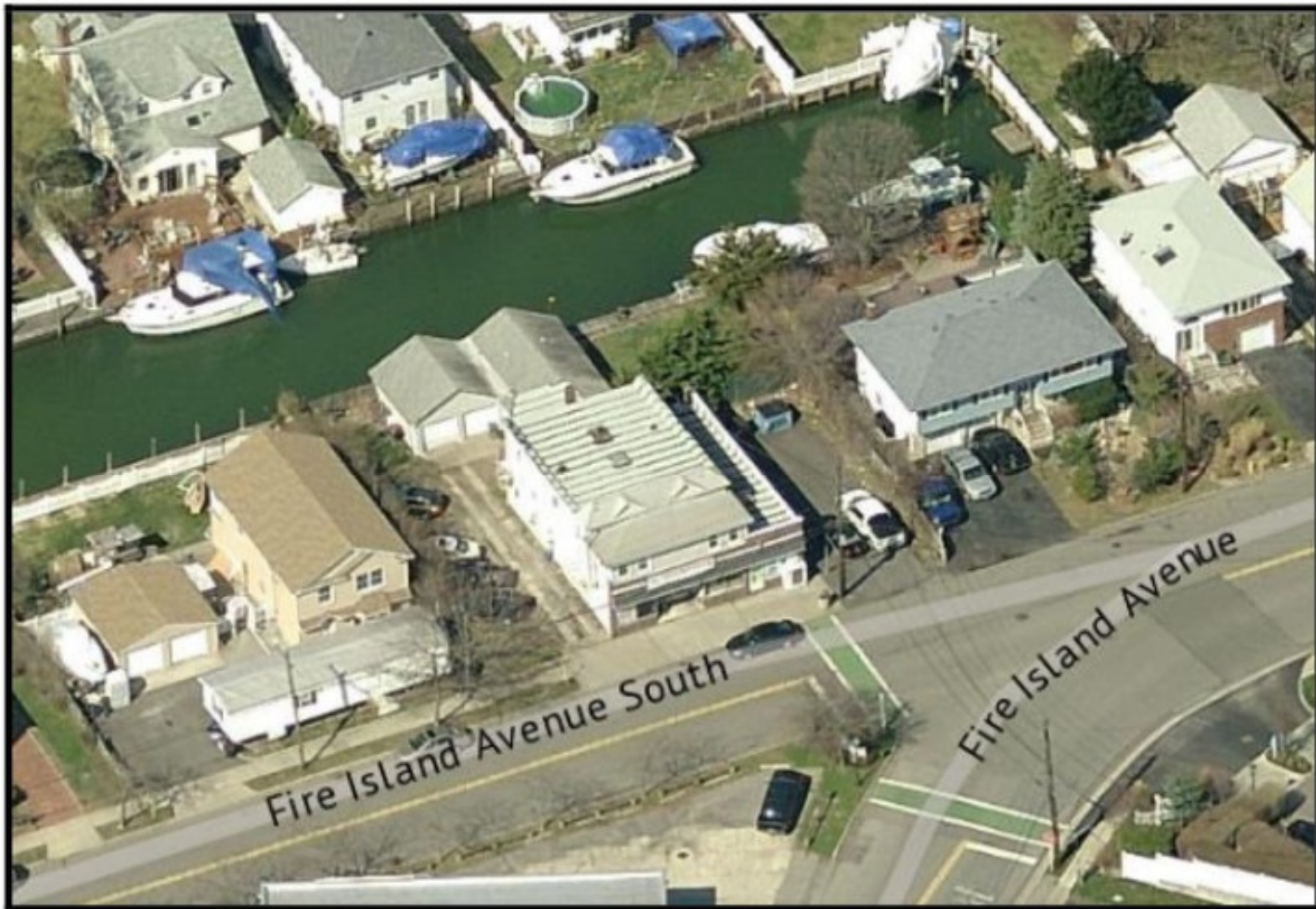
AERIAL VIEW FACING WEST TOWARD FRONT OF SUBJECT
