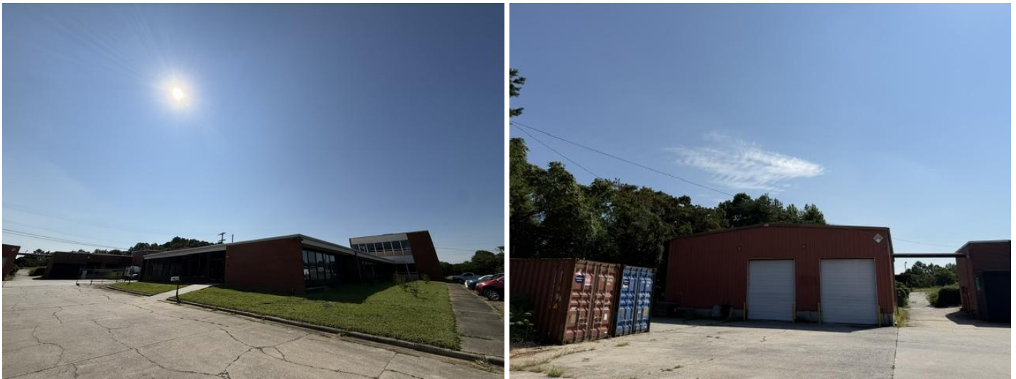
Left: Street-front façade — brick & glass, excellent street presence. Right: Rear loading court — paved, truck-accessible, ample maneuvering room.
