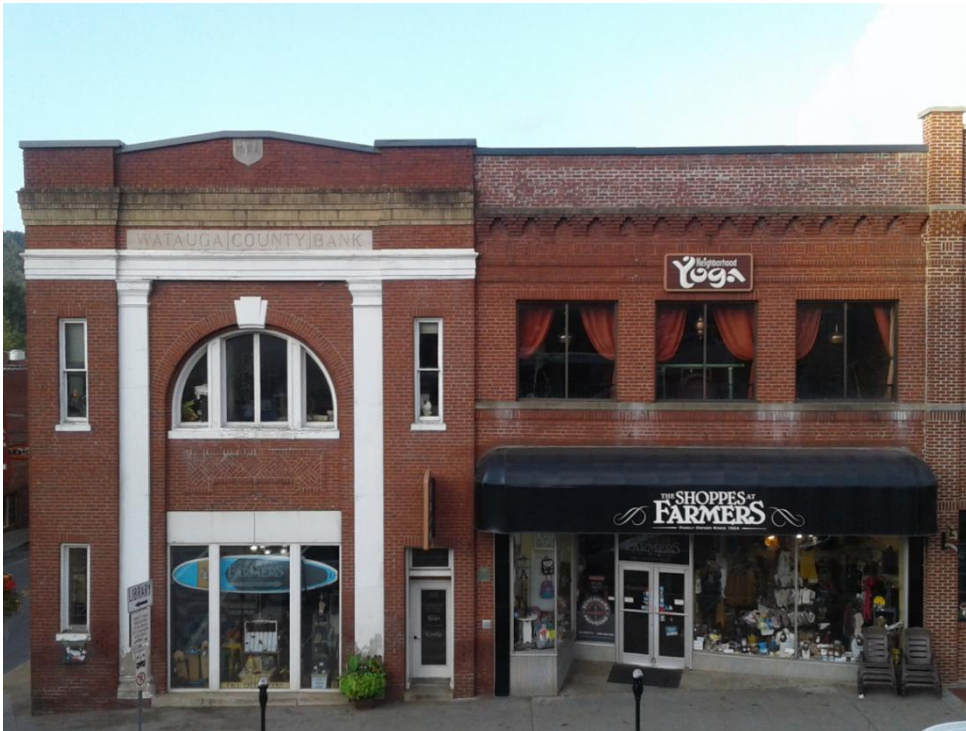
Graphic 14.19.06-7 Desired Downtown Design 671 West King Street Identified Features: Building demonstrates sympathetic renovation with brick materials, brick detailing, fenestration percentages, transoms over doors and awnings
