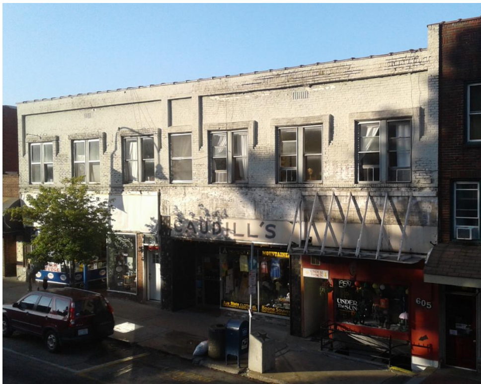
Graphic 14.19.06-3 Desired Downtown Design: 607 West King Street Identified Features: Original brick materials, brick detailing and coping; fenestration percentages; transom over door
