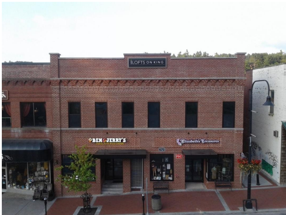
Graphic 14.19.06-7 Desired Downtown Design 671 West King Street Identified Features: Building demonstrates sympathetic renovation with brick materials, brick detailing, fenestration percentages, transoms over doors and awnings
