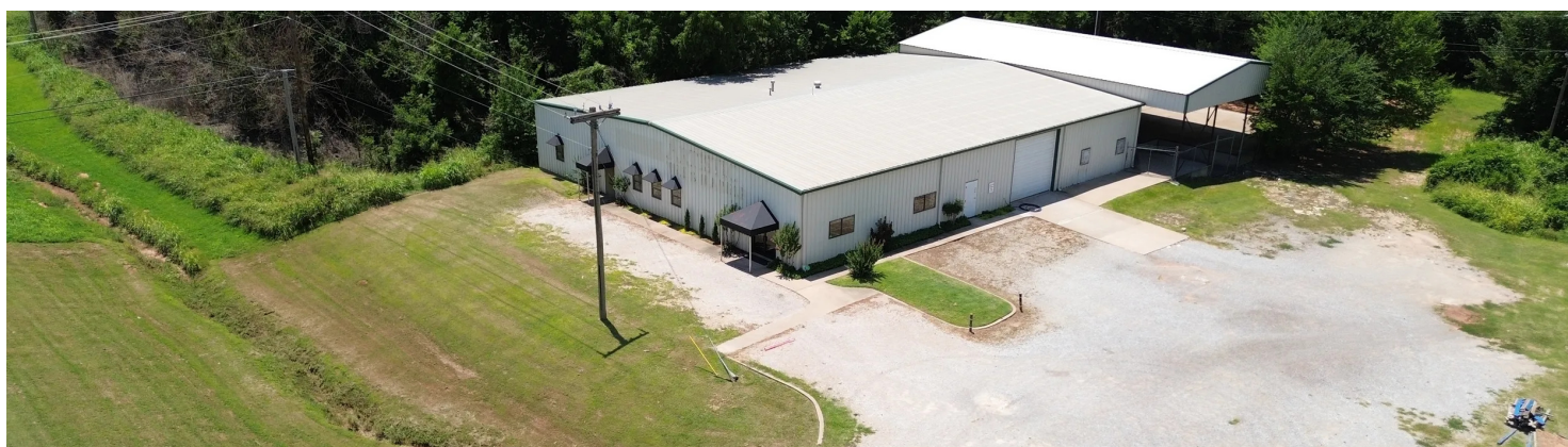
LOOKING SOUTH WEST
