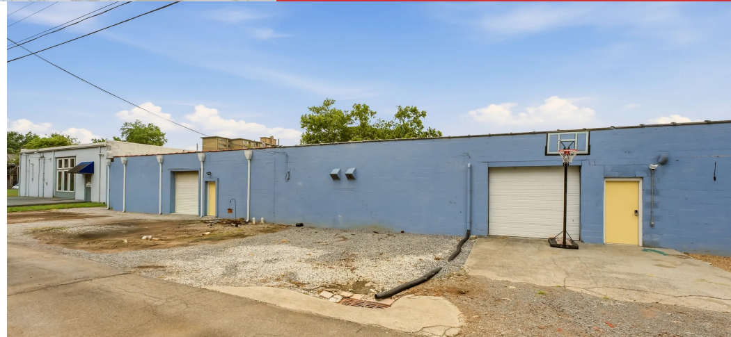
Rear Exterior- Four Grade Level Drive In Doors
