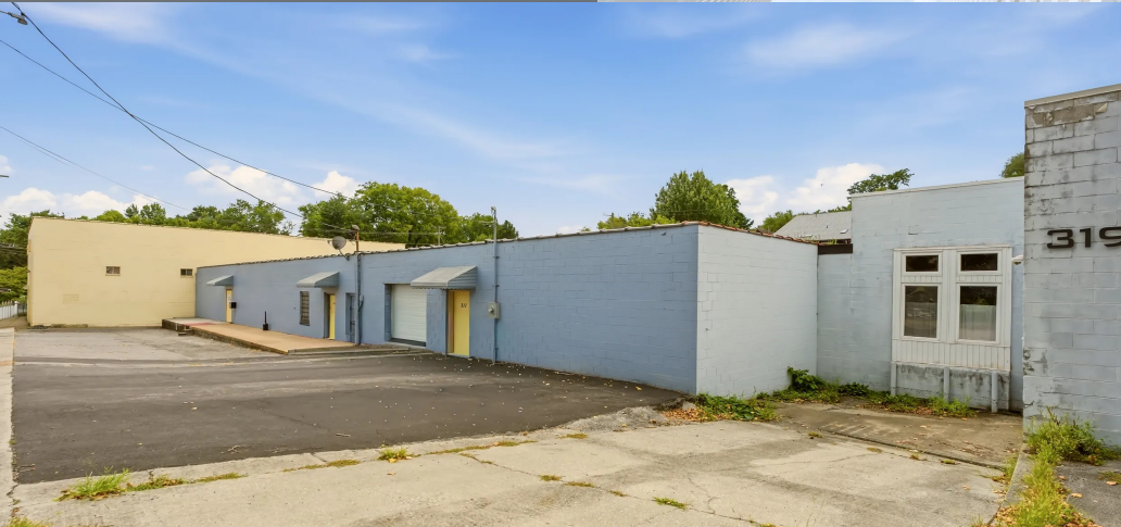
Front Exterior- One Grade Level Drive in Door
