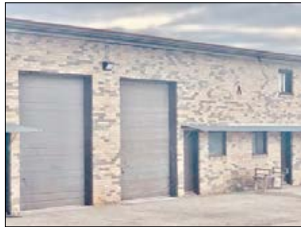
Dock High Doors C7 & C8
